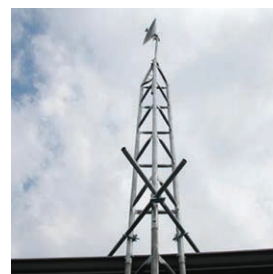
Install segments to reach up to 12.24 metres
