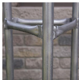
Double bead welded 18-gauge galvanized steel
